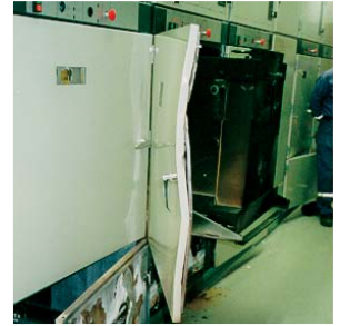
Traditional protection relay systems do not provide fast enough protection in an arc-fault situations.
