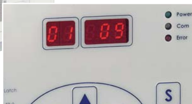
A detailed address code of the fault location is displayed on the central unit.
