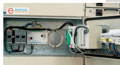
I/O units are mounted in the apparatus compartment. Connection to central unit is made with a modular cable.
